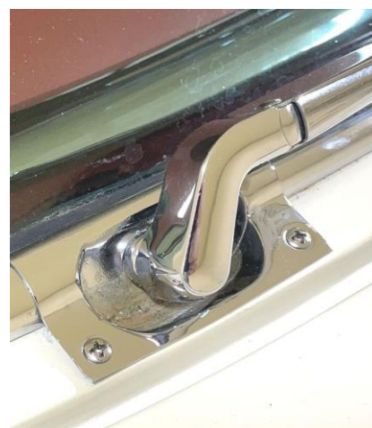
Later style; no front fold, screws sit exposed on top
